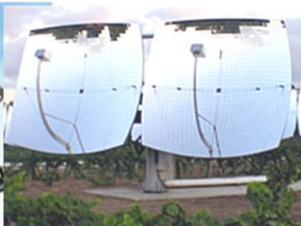
Hybrid collectors capture the heat energy from the sun that is otherwise lost by flat plate photovoltaic panels. They do it with mirrors. Mirrors reflect sunlight into an absorber when photovoltaic (PV) cells first convert a portion to electricity. Coolant running through the absorber cools the PV cells and captures the heat portion of the sun's energy as a hot fluid.
